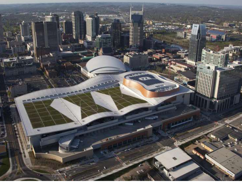
Music City Center and its green roof
